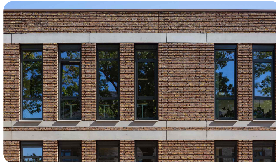
Horizontale geleding in gevel
